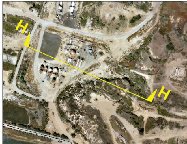
Aerial Photograph of Existing Conditions
